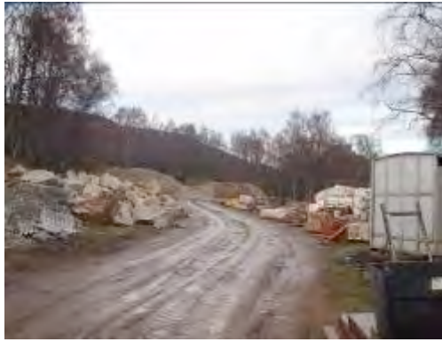
Fig. 6 - Further area of stores, plant and materials
